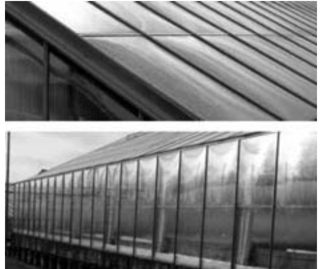
Fig. 3: Details of the roof and wall area with the G/F cover
