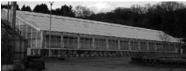
Fig. 2: Greenhouse compartment with the glass foil combination on roof and wall area
